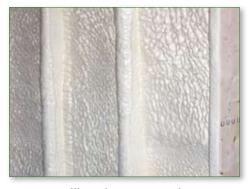
gypsum wallboard or an equivalent 15-minute thermal barrier complying with, and installed in accordance with, IBC Section 2603.4 or IRC Section 316.4 as applicable, except when installed in attics and crawlspaces. The maximum thickness of the insulation is 7" (192.5 mm) in the walls and 11.5" (292.1 mm) in the ceiling.
