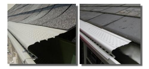
**The Leaf Techus** has a very unique feature. It consists of a built-in hood and louvers. This is the most effective gutter cover system in the market.
