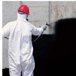
**A** The TUFF-N-DRI flexible waterproofing membrane is spray-applied to bridge foundation settling cracks and reliably guard against water penetration through basement walls. Local Barrier Solutions Contractors install the membrane for consistent application coverage and thickness.
