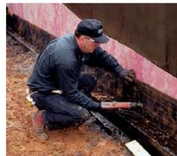
As an option, DrainStar® Stripdrain can be added to your TUFF-N-DRI installation. DrainStar collects and moves water away from the foundation, and can replace the hassles of traditional drain tile and gravel.
