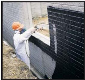
Your local Barrier Solutions Contractor skillfully spray-applies WATCHDOG WATERPROOFING for seamless, consistent protection against moisture.
